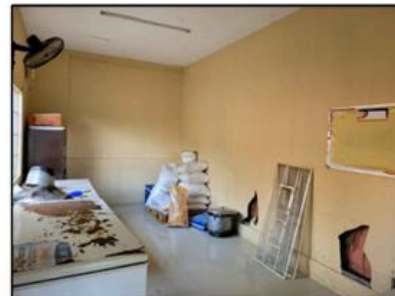
EXISTING KITCHEN STORAGE
