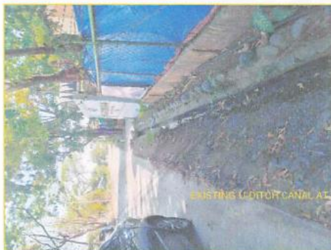
EXISTING U-DITCH CANAL AT RIGHT SIDE TO BE DEMOLISHED
